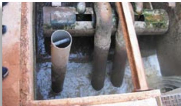
Batch feeding siphon in empty chamber, constructed wetland, Roussillon, France
